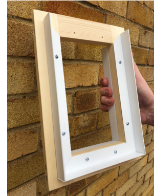
Angles with internal legs/screws
